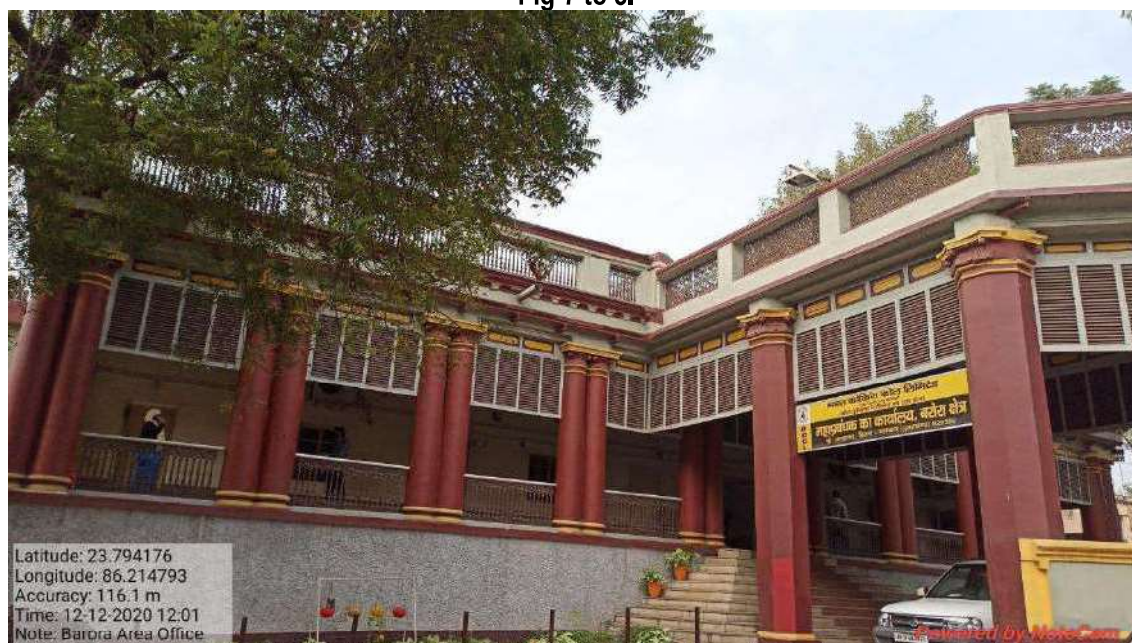
Proposed Rain Water Harvesting Site – Barora Area Office, Cluster-I, Barora Area
